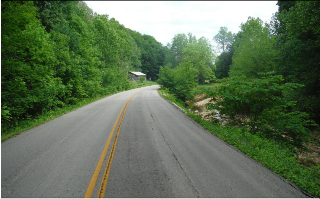
Slope/shoulder stability issues adjacent to the roadway at Buck Crawford Place at Indian Creek. 5/20/2015
