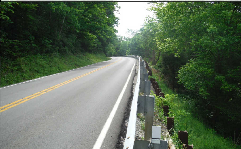
Location 4: KY 344 MP 14.30 to MP 14.40
