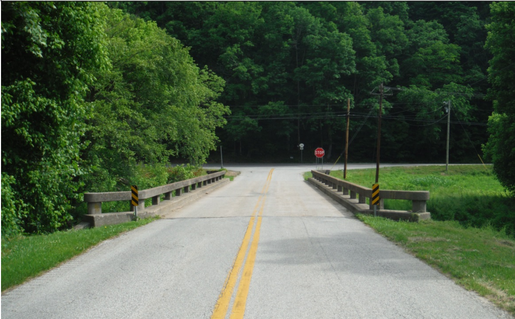
Location 5: KY 344 / KY 377 Intersection
